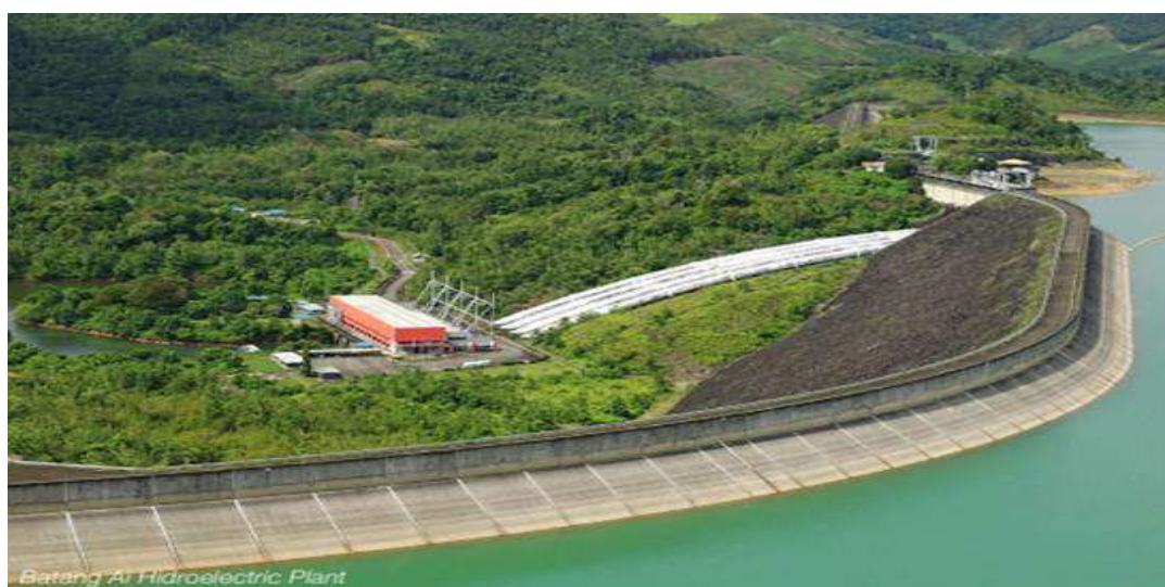
Figure 4-25: Batang Ai Dam
