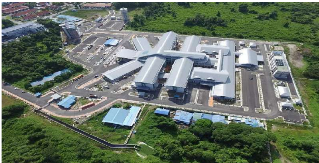
Figure 4-54: New Hospital in Sri Aman under construction
