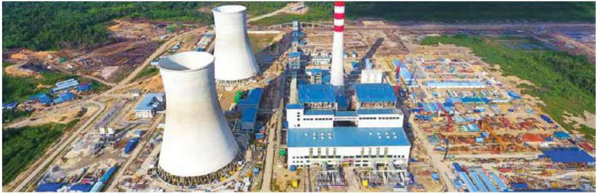
Figure 4-18: Balingian Coal-Fired Power Plant in Mukah, Sarawak
