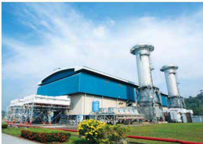
The 317MW Bintulu Combined Cycle Power Station.
