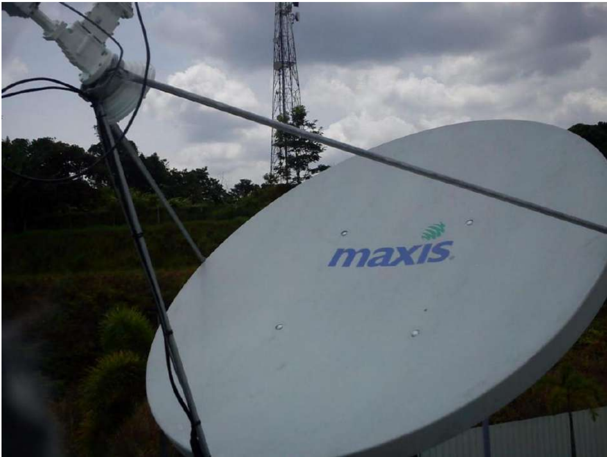
Figure 4-44: An Example of VSAT Dish Antenna from Maxis
